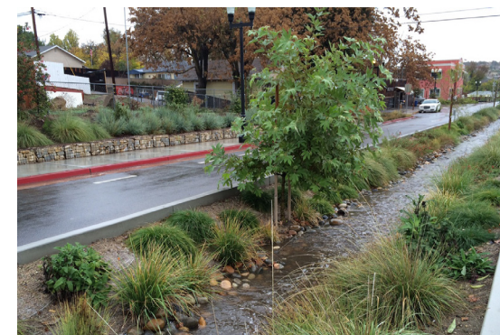
D: TREE TRENCH A Tree trenches are encouraged to be located between the public road and public sidewalk. In low-density residential or in areas without adjacent parking, the tree trenches will be designed to maximize growing area and stormwater volume.
