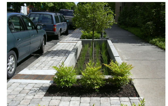
D: TREE TRENCH B Tree trenches are encouraged to be located between the public road and public sidewalk in the neighborhood node. In areas adjacent to higher density residential development and/or in areas with adjacent parking, the tree trenches will be designed to support safe pedestrian circulation.
